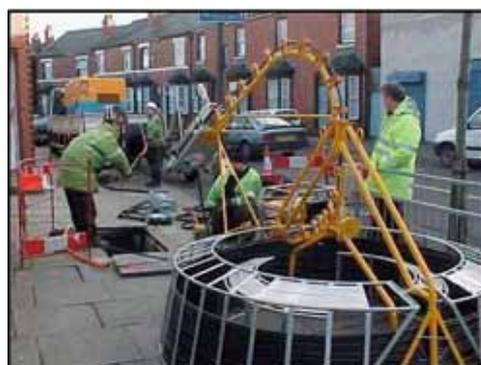
Figure 43: Deploying duct infrastructure.
