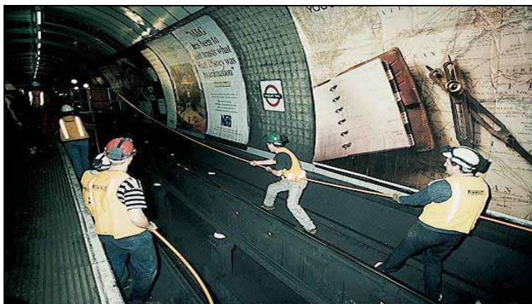
Figure 80: Cable installation in a train tunnel.
