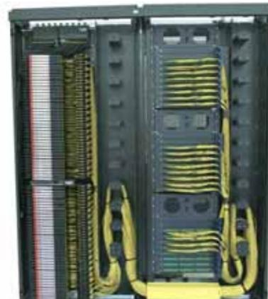
Figure 12: High density fibre management.
