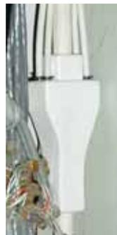
Figure 40: Branching unit without splicing.
