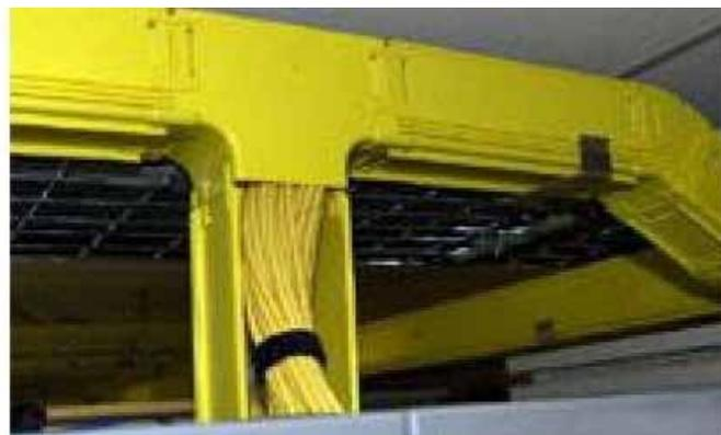
Figure 92: Examples of overhead cable guiding systems.
