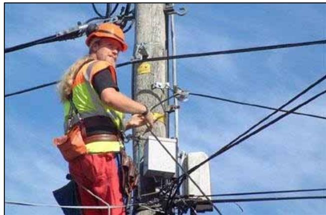
Figure 72: Aerial cable installation.
