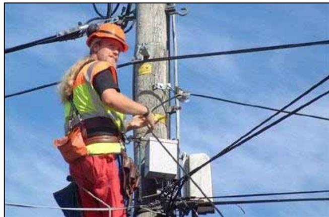
Figure 72: Aerial cable installation.
