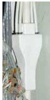
Figure 40: Branching unit without splicing.
