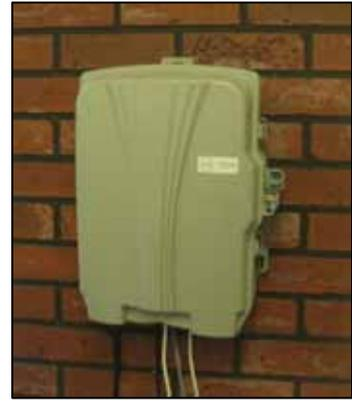
Figure 85: External fibre termination box.
